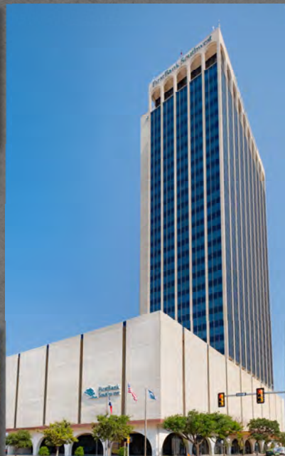
FIRSTBANK SOUTHWEST TOWER 600 S Tyler
