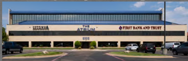
THE ATRIUM AT COULTER RIDGE 6900 I-40 West
